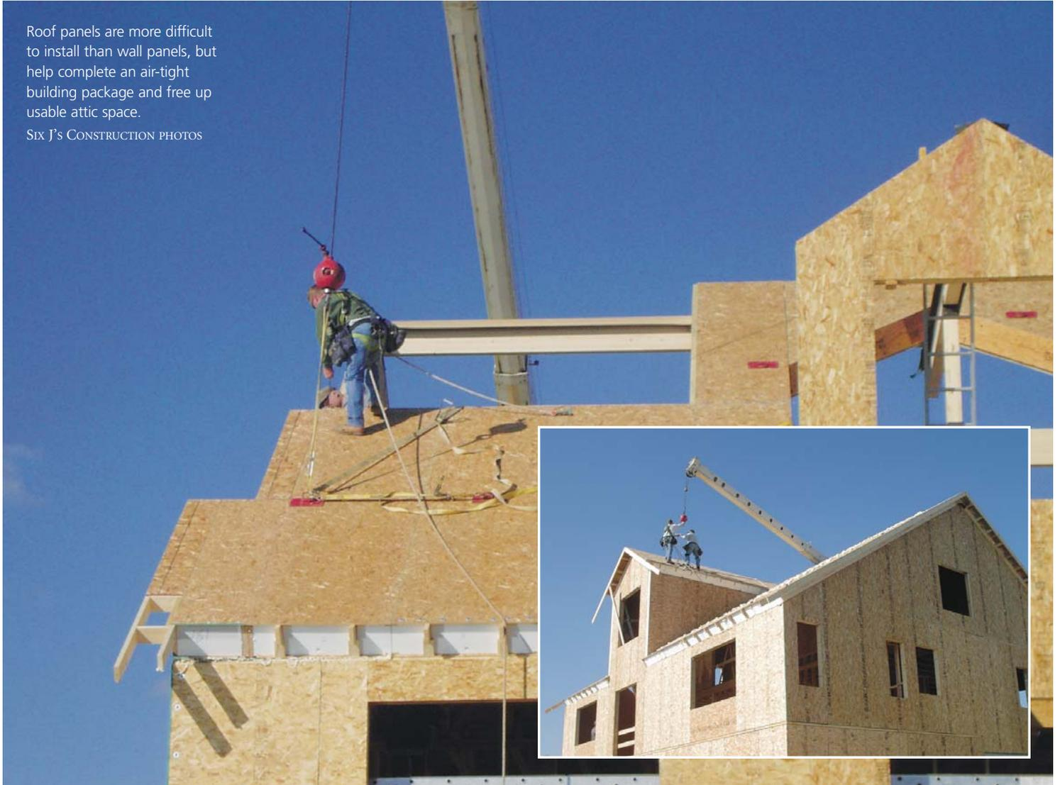
of the time he has to trim a panel when he gets to a corner, and recess the foam back out. "It's the hardest thing to get a hold of, and you're only 1/2, 3/8 inches off," he says. "And roofs are tricky for an everyday framer." SIPs builders also use special tools like ratchet straps, which allow installers to gradually move panels into position without using blunt force that could damage the foam or OSB.
