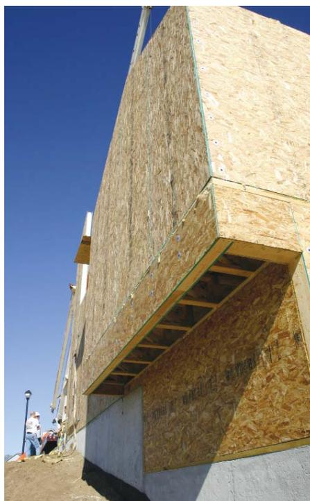
The builders involved in Energy House say cantilevers such as this are easier to build with SIPs than with stick framing.
